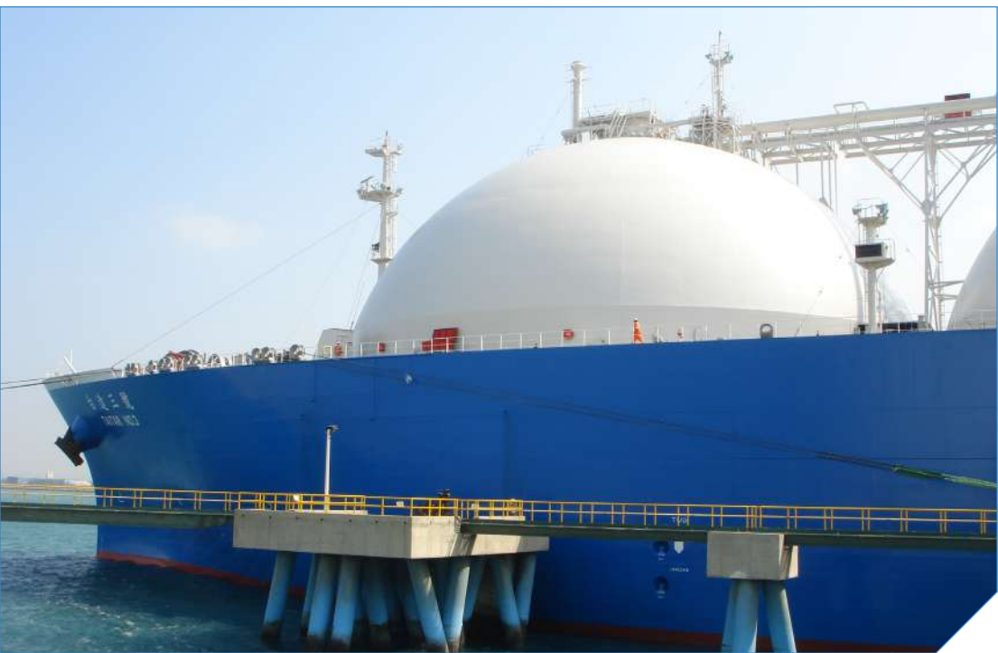
CPC Corporation LNG Taichung Receiving Station
