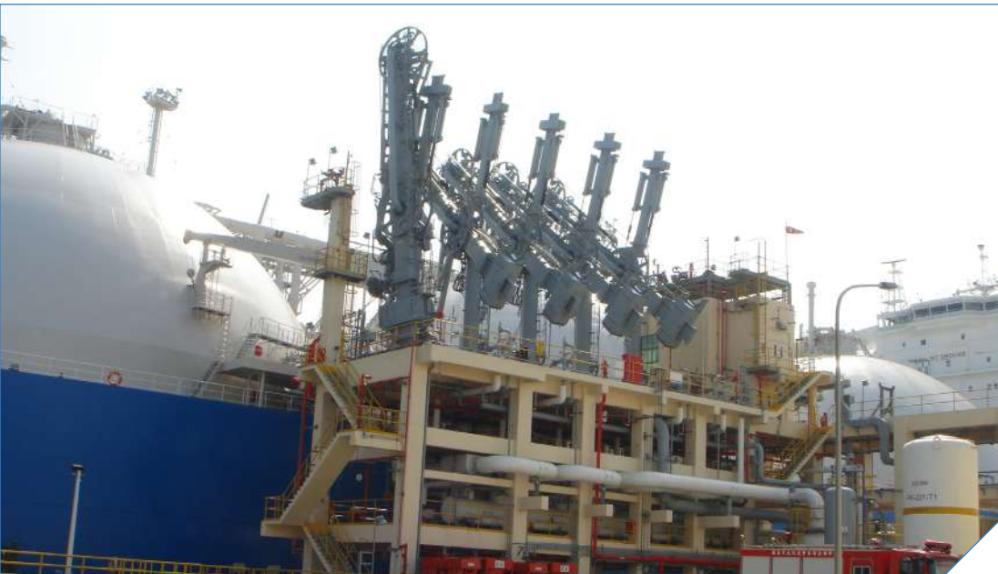
CPC Corporation LNG Taichung Receiving Station
